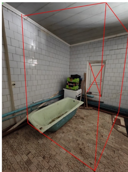
Photo 17 Space for sanitary block for staff
