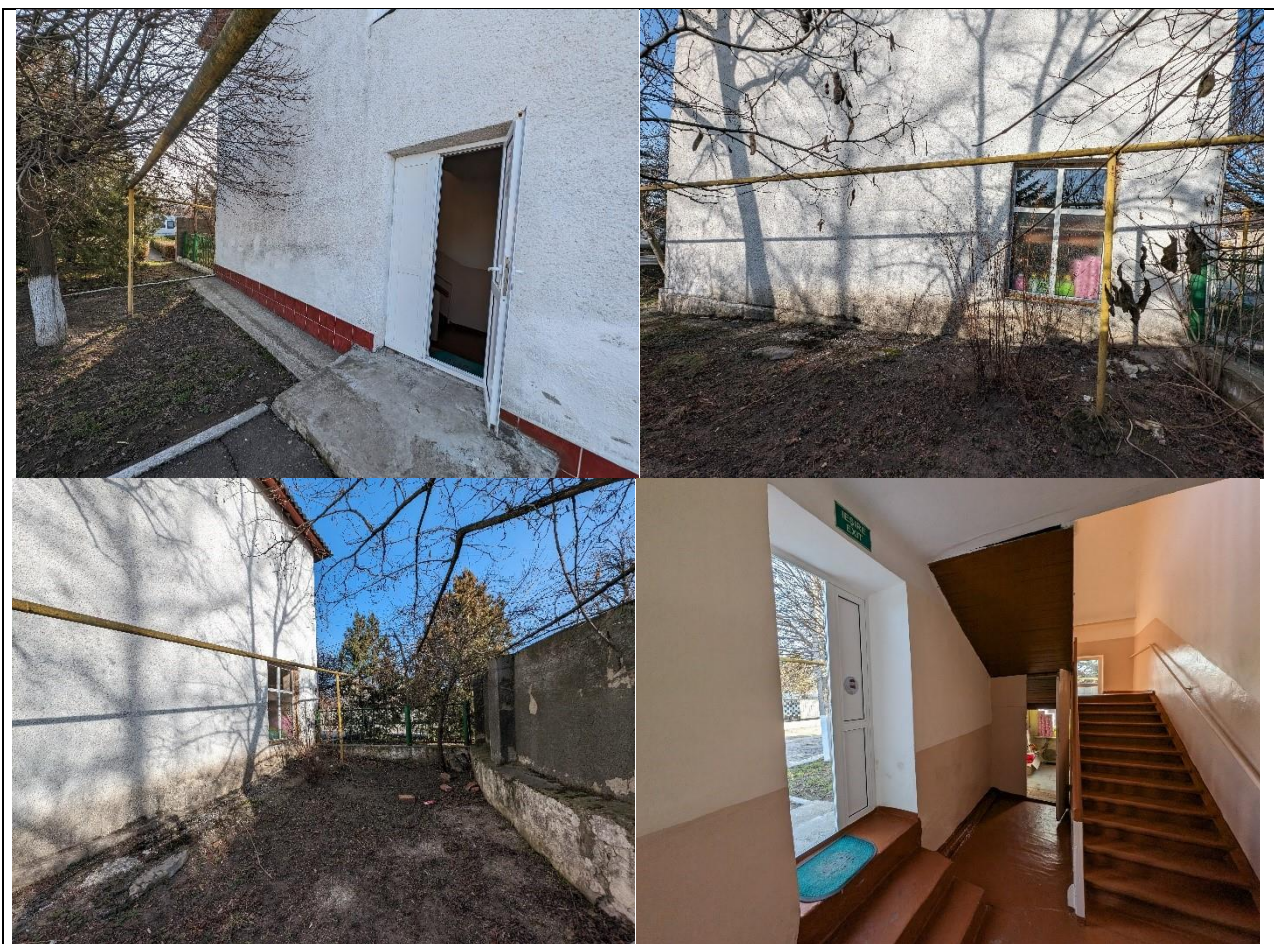
Proposed place for location of the new annex for accommodation of additional WASH facilities
