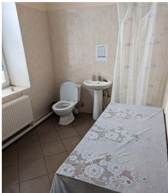
Photo 6 Proposed space for the annex
