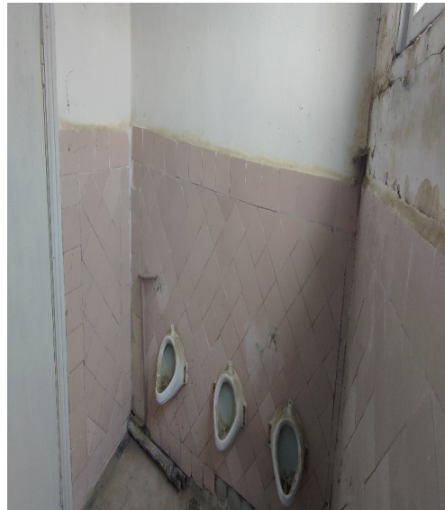
Block C, GTS Level 3 left
