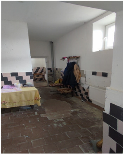
GTS level 2 Block D, shower/toilet
