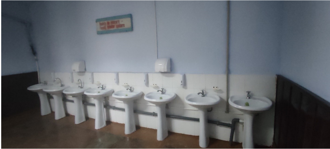
Install hand washing – canteen access
