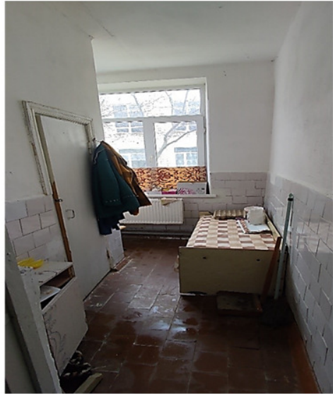
GTS Level 1 Block C
