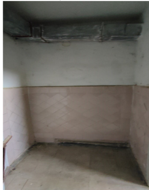
Block C, GTS Level 3 left
