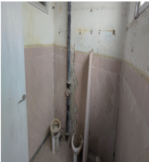
Block C, GTS Level 3 right
