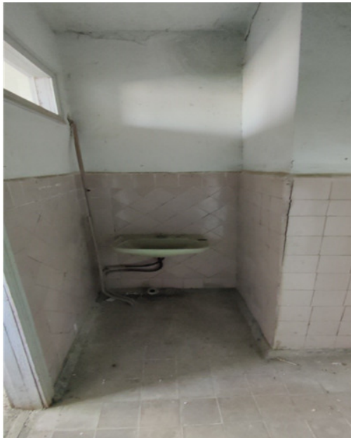
Block C, GTS Level 3 left
