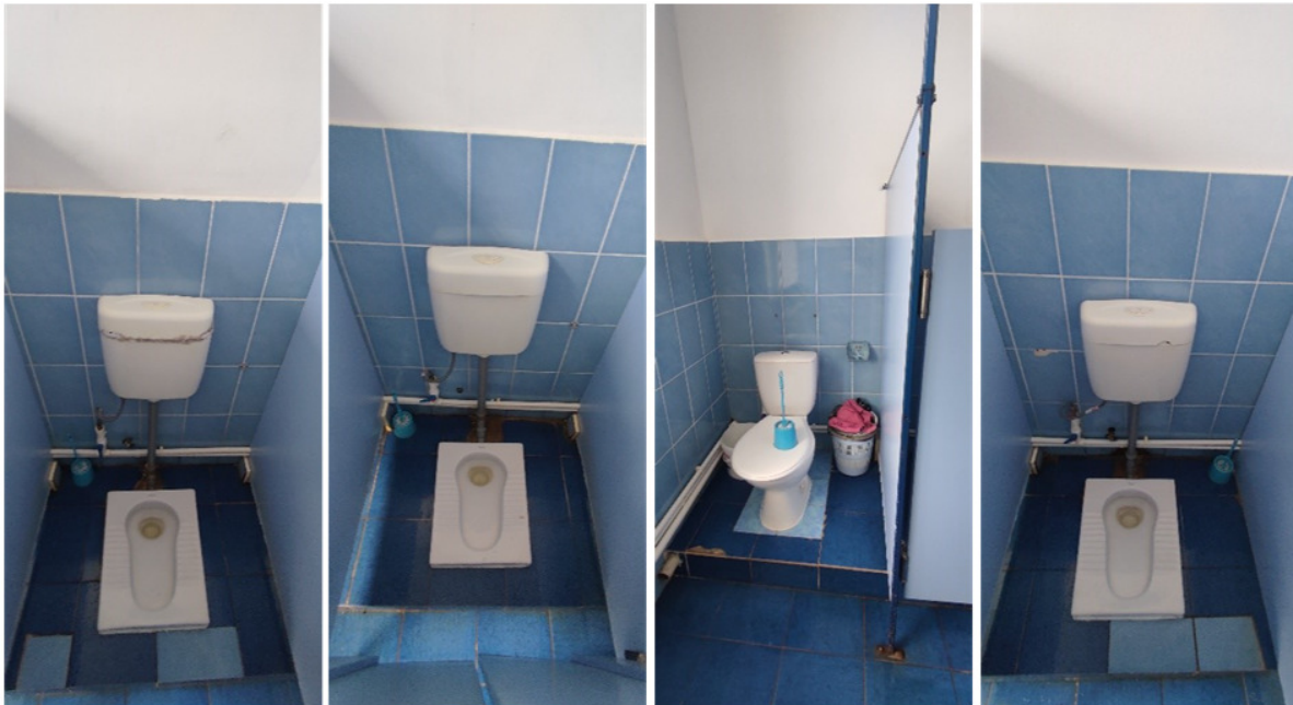
GTS level 1 on the right
