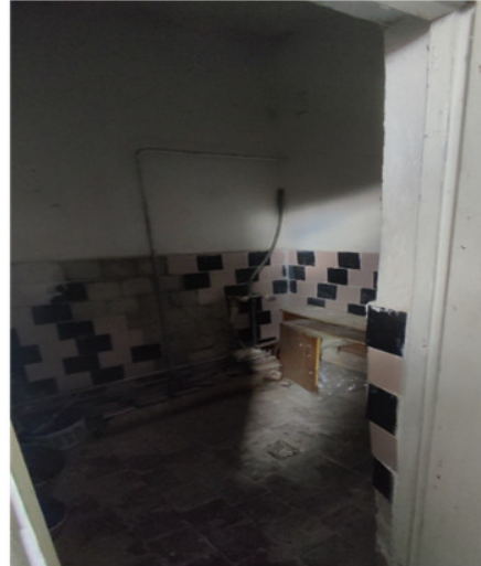
GTS level 2 Block D, shower/toilet
