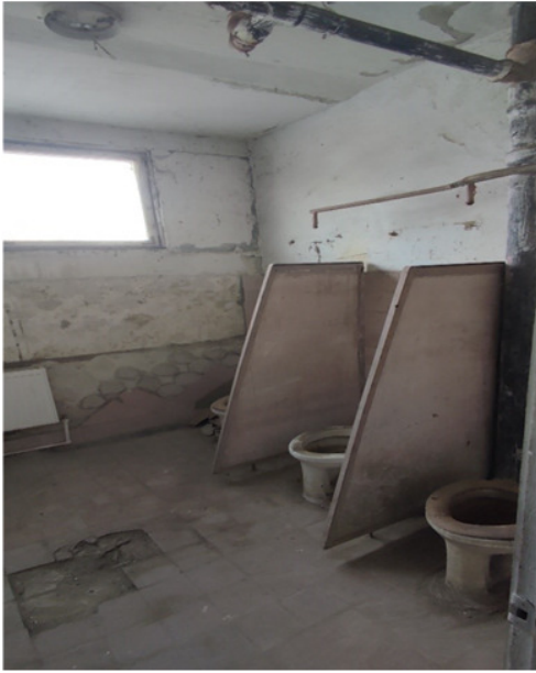
Block C, GTS Level 2 right
