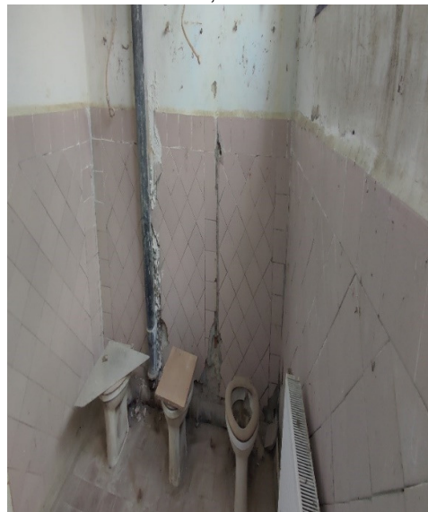
Block C, GTS Level 2 left
