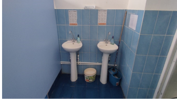
GTS level 1 on the right
