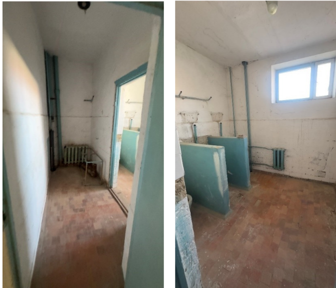
Camera for boys GTS, level 3, block A.
