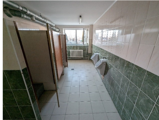
GTS guys, necessary changing doors and rehabilitation of the ventilation system
