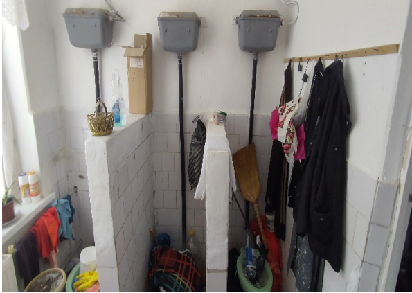
GTS Level 1 Block D
