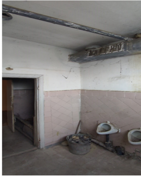
Block C, GTS Level 2 right
