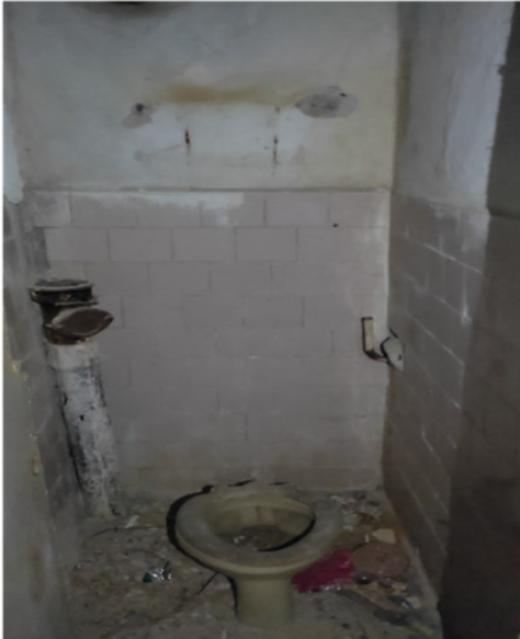
GTS boys locker room
