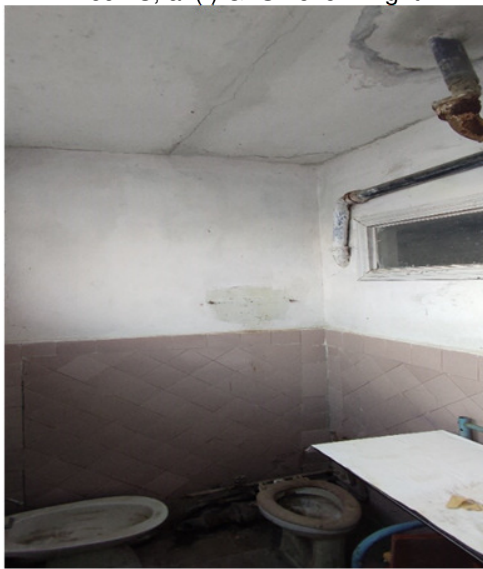
Block C, GTS Level 1 left
