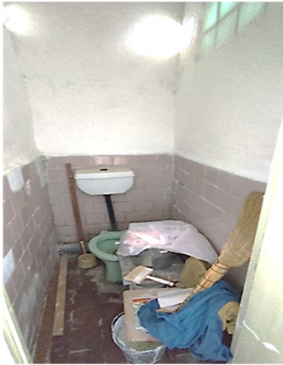
GTS Level 1 Block C
