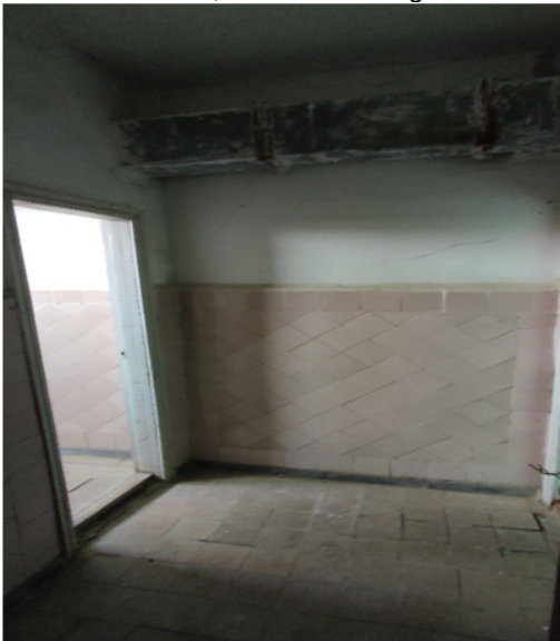
Block C, GTS Level 3 right
