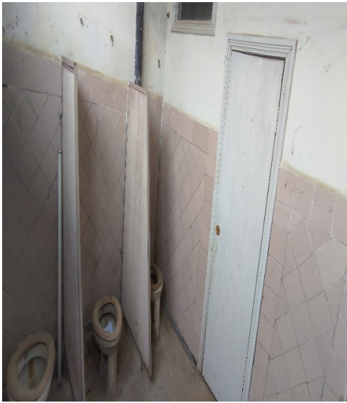
Block C, GTS Level 3 left
