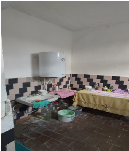
GTS level 2 Block D, shower/toilet
