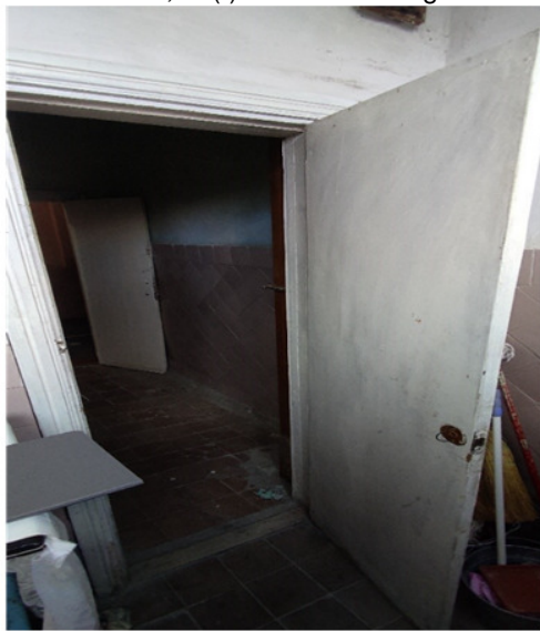
Block C, GTS Level 1 left
