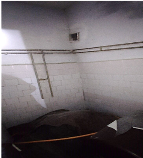
Boys locker room, level 2
