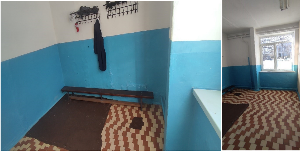
GTS boys locker room
