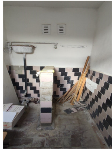
GTS level 2 Block D, shower/toilet
