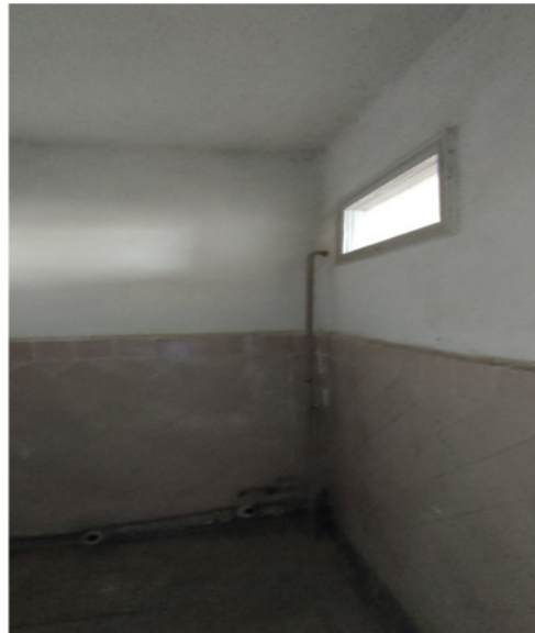
Block C, GTS Level 3 right
