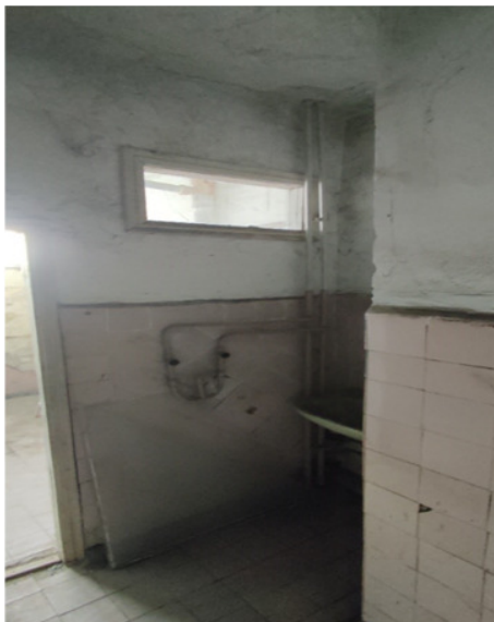
Block C, GTS Level 2 left
