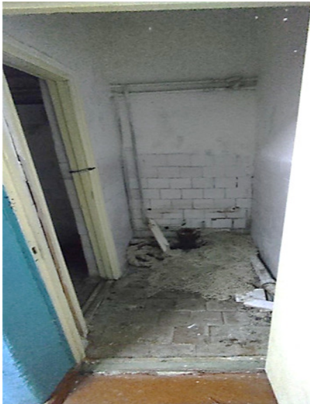
Boys locker room, level 1
