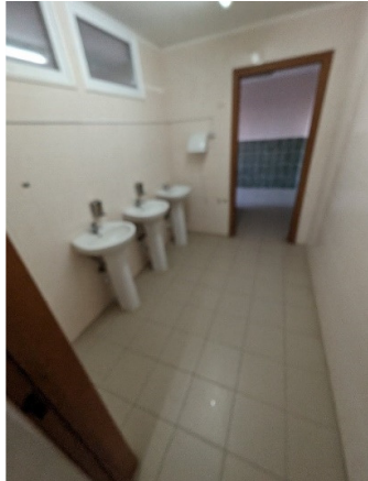
GTS guys, necessary changing doors and rehabilitation of the ventilation system
