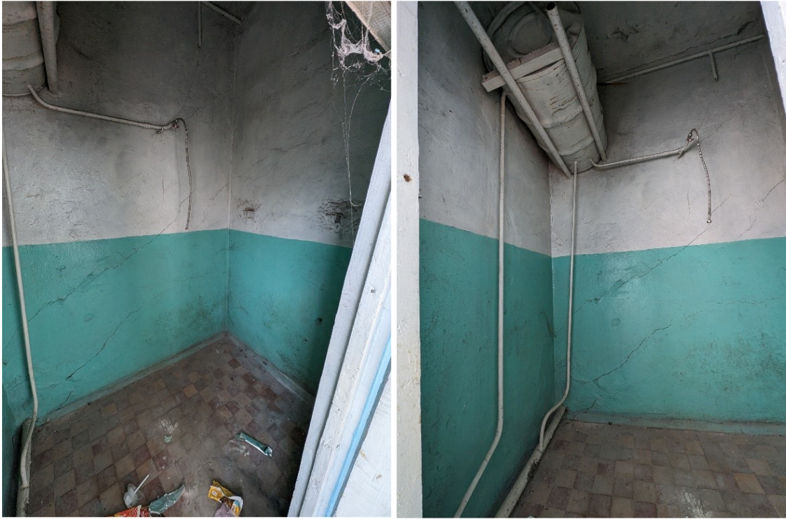
Sports hall shower room boys
