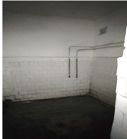
Boys locker room, level 1
