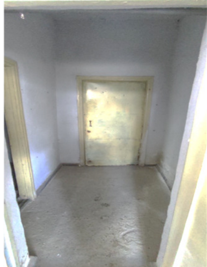
GTS Level 1 Block B
