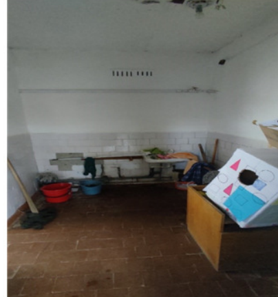
GTS Level 1 Block D
