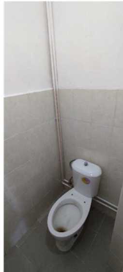
GTS boys locker room
