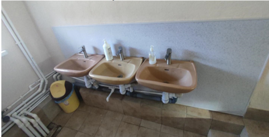
Cafeteria access area, toilet washing facilities
