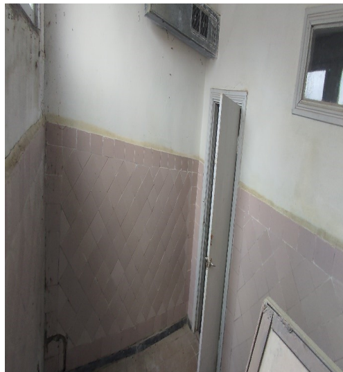
Block C, GTS Level 3 right
