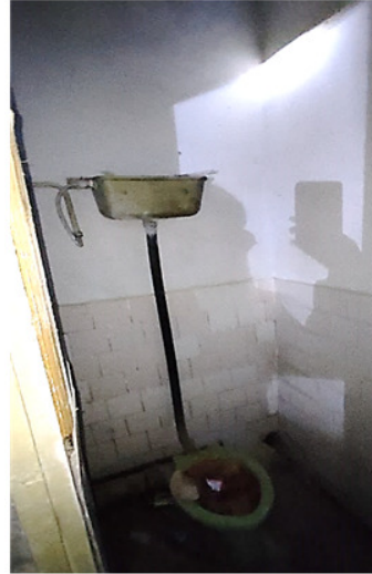
Boys locker room, level 2
