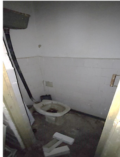
GTS Level 1 Block B
