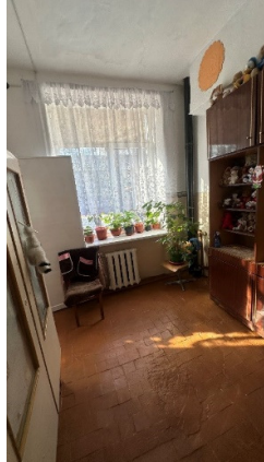
Current situation toilet for girls, level 2.
