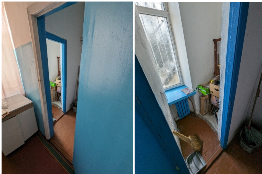
SG for kitchen staff – construction of sanitary groups for staff, with all internal facilities and service systems
