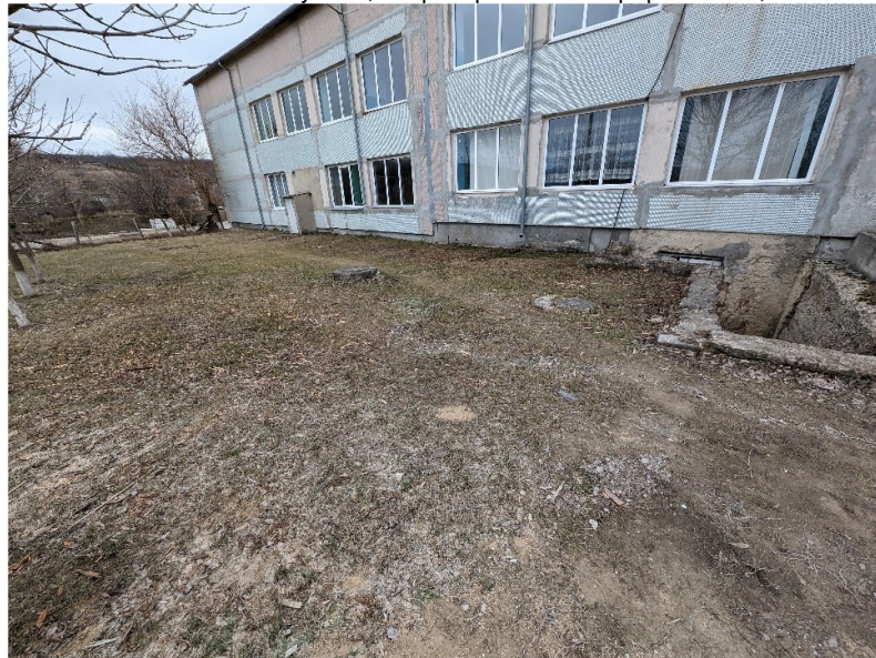
The cesspool-locality does not have a centralized drinking water system, at the moment the institution is supplied from the spring, it is proposed to design and build an artesian well and water tower
