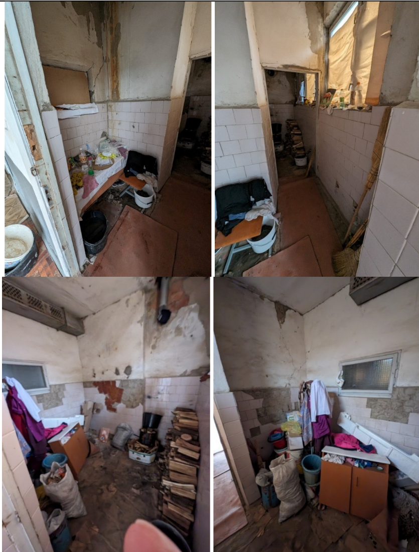
Block B, 2nd floor – SG renovation for boys 5-9 class
