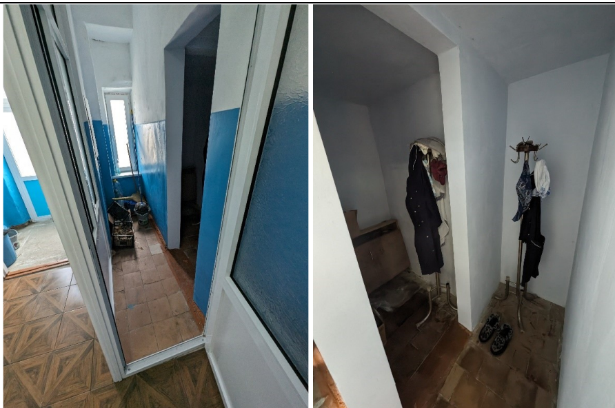
Cafeteria entrance – construction of SG and showers for staff
