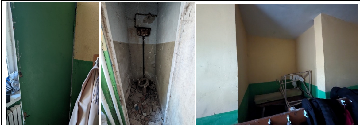
Sports hall – construction of showers and SG for boys
