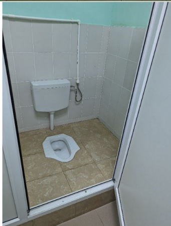
GTS guys-required Ventilation system and hand dryer, lack of centralized water
