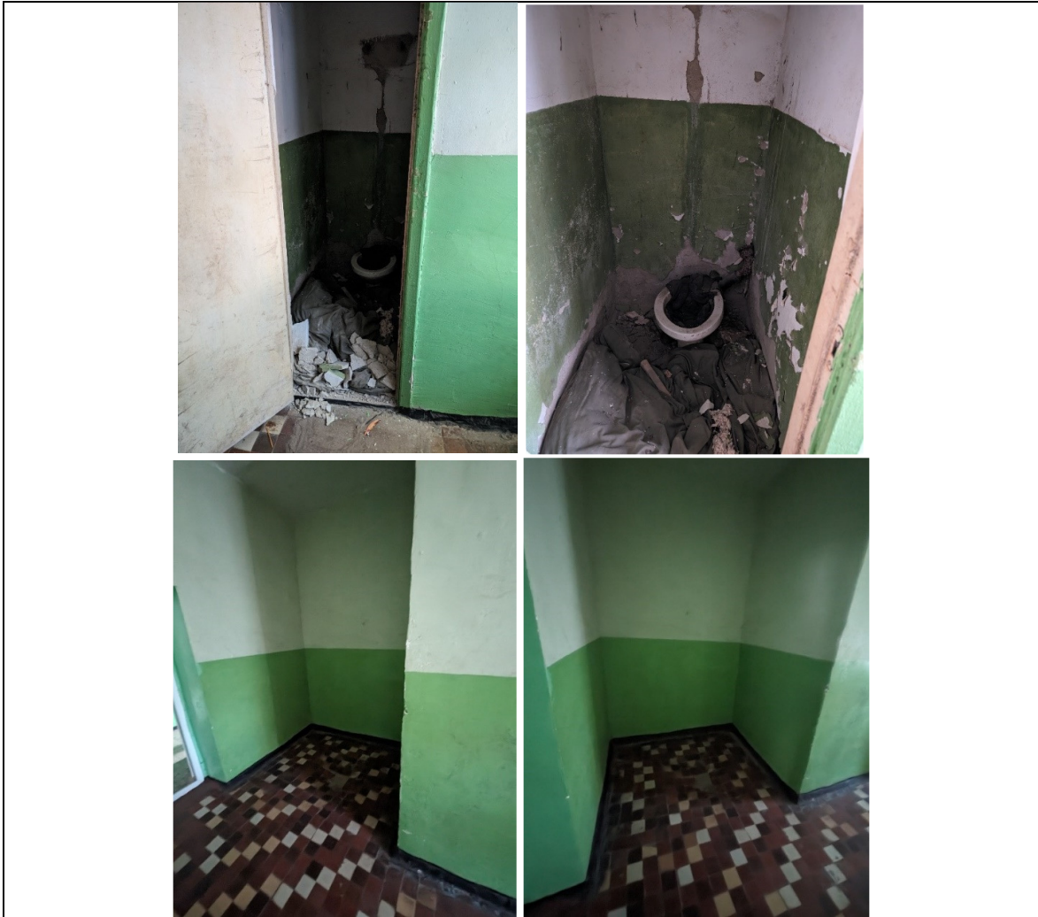
Sports hall – construction of showers and SG for boys
